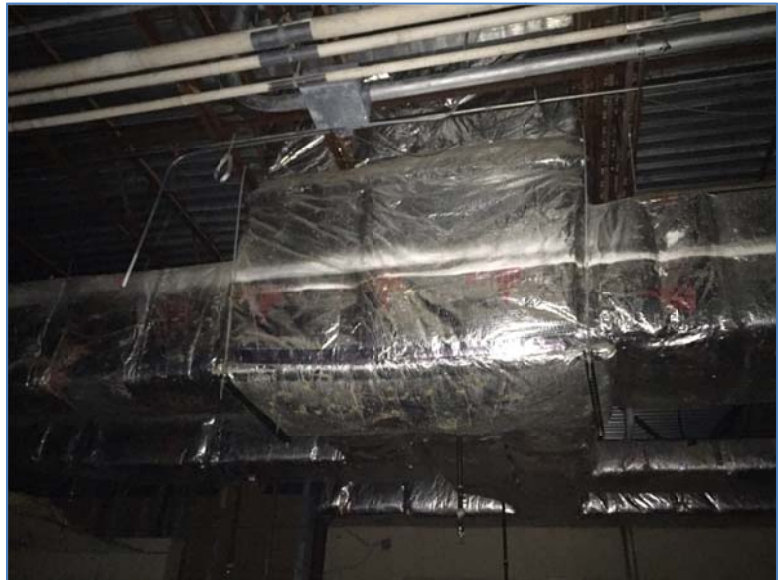
Existing exterior wrap ductwork noted above existing ceiling.
