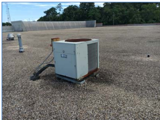
Existing split system condensing unit on rooftop.
